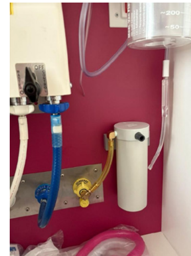
Figure 5. The Bassoon-style scavenging setup in birth suite at Flinders Medical Centre, South Australia
